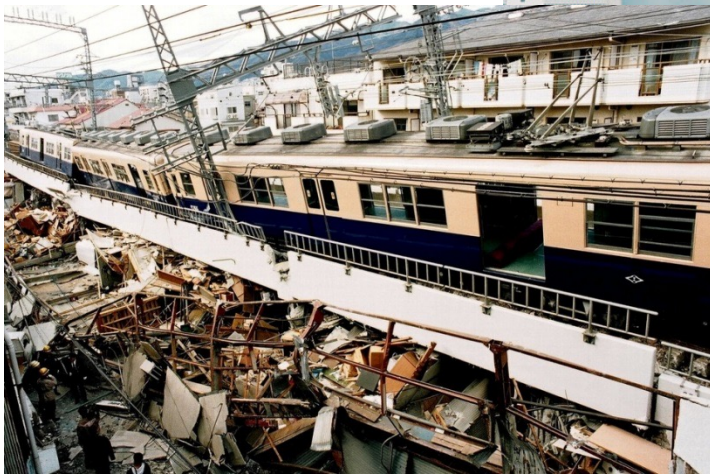
Damaged railway track
