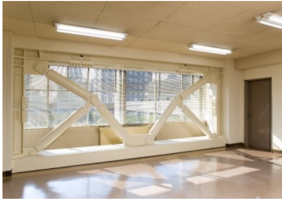
Seismic Brace with vibration damper inserted.
