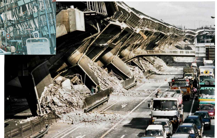
Collapsed viaducts of an expressway
