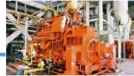
Power generation using digestion gas
