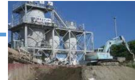
Improved soil for backfill
