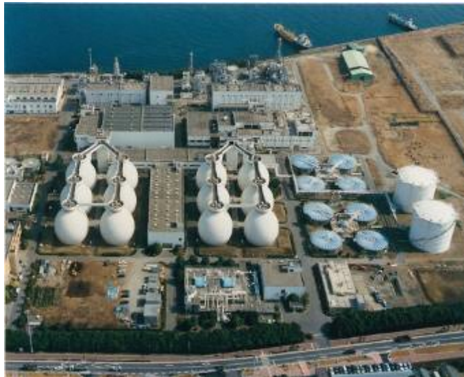
Sludge treatment center
