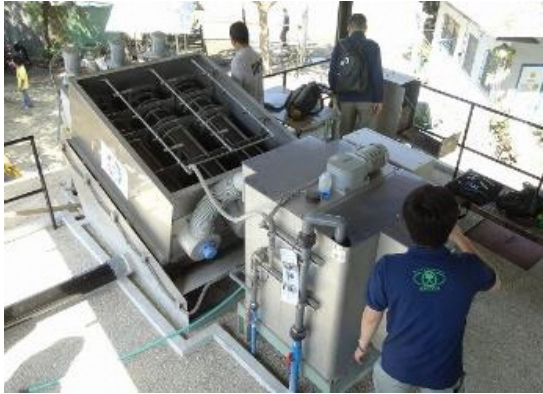
JICA support for Japanese SMEs' overseas business development (Demonstration test of sludge dewatering system by Amcon Inc., a Yokohama-based SME)
