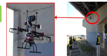
Inspection of infrastructure using drones
