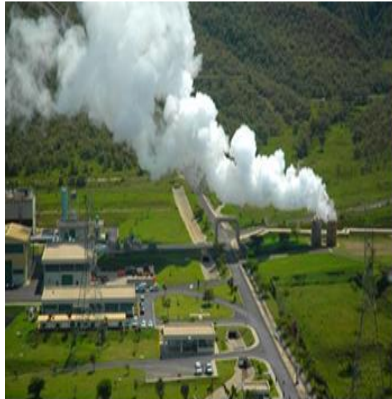
Green Energy to Power our Nation – Ol-Karia Geothermal plant
